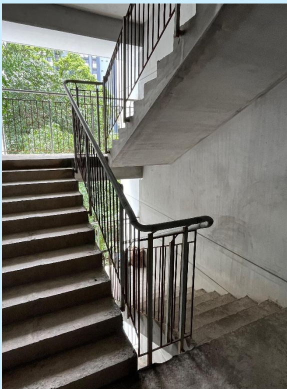
T1 FIRE STAIR G.I HANDRAIL
