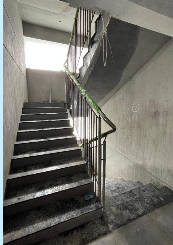
T1 GRANITE FLOORING & SS HANDRAIL WORK
