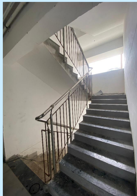
T1 S.S HANDRAIL WORK
