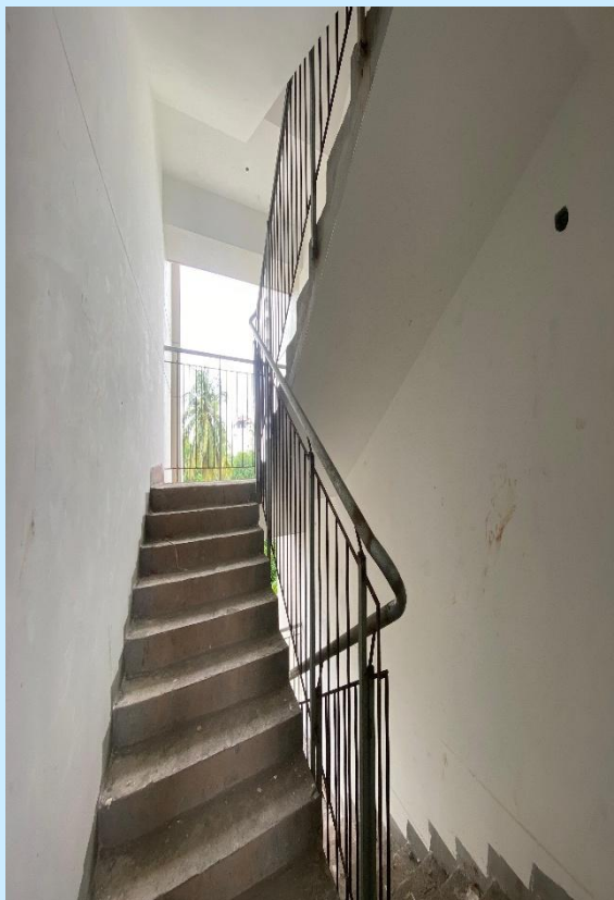
T1 FIRE STAIR G.I HANDRAIL
