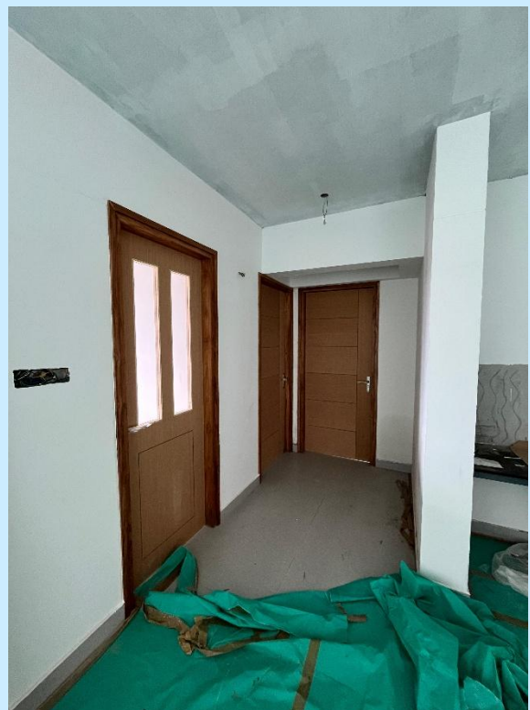
T1 4 TH FLOOR DOOR FIXING
